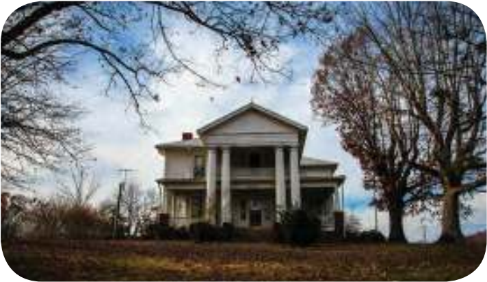
Single-family homes, such as this farmhouse, are the primary land use type found within the low-density growth sector of Stokes County.
